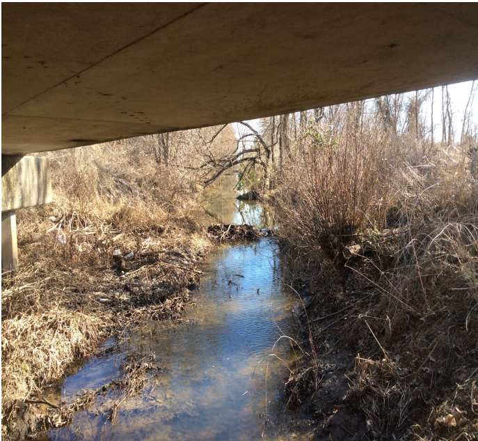
PHOTO 1 Description Right side of bridge has small beaver dam blocking channel.
