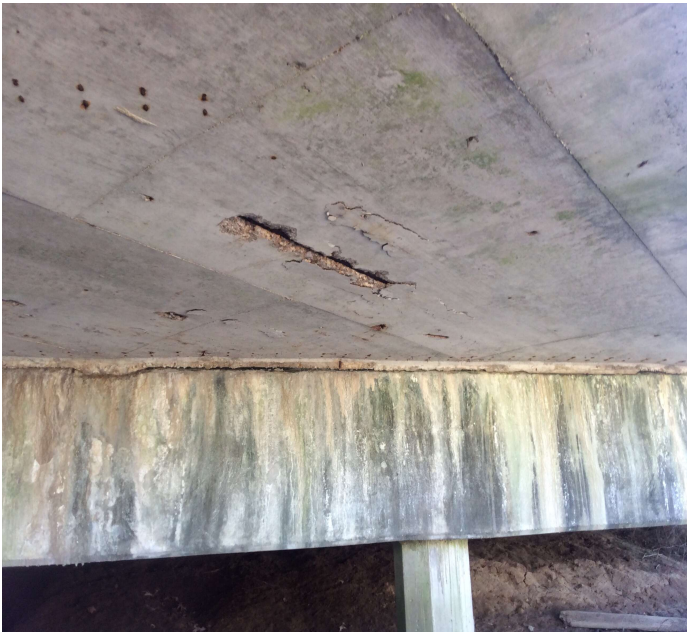
PHOTO 1 Description Spall in soffit span #2 left side.
