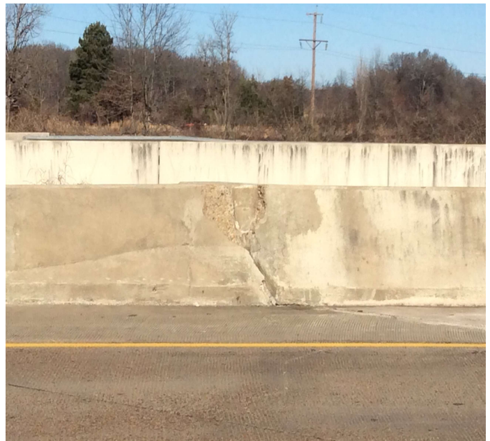
PHOTO 2 Description Abutment #1 left rail spall.
